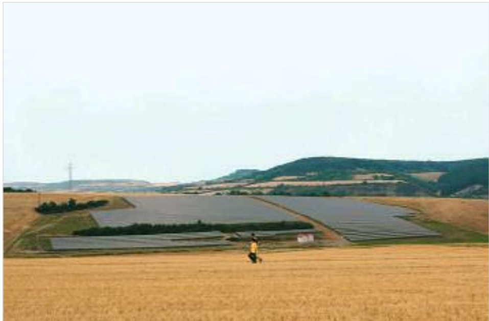
Laudenschbach Solar Park, 809 kWp
