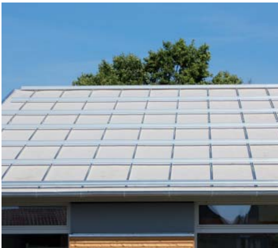
Figures 1 and 2: Roof with an installed water-bearing layer and the Phoenix TectoSmart mounting system
