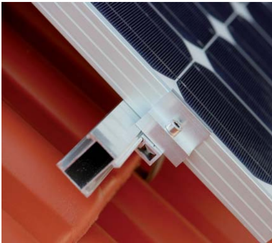
Figure 13: Module with module end clamp set
