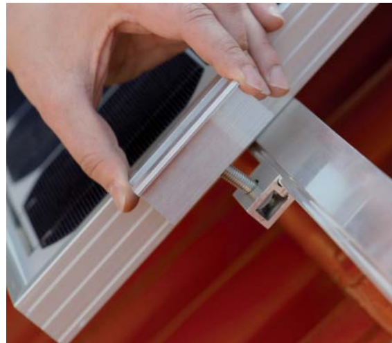
Figure 14: Module with module middle clamp set
