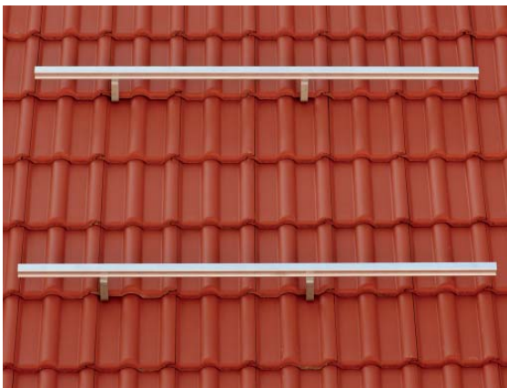
Figure 7: Aligning the rail using a tension string
