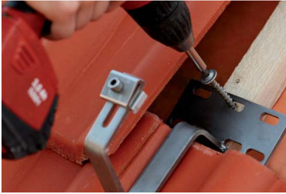
Figure 3: Screwing the roof hook tight
