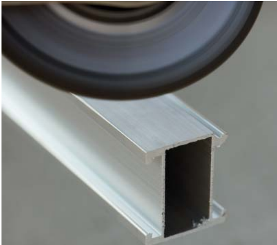
Figure 5: Cutting the rail to length
