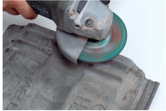
Figure 4: Modifying the roof tile
